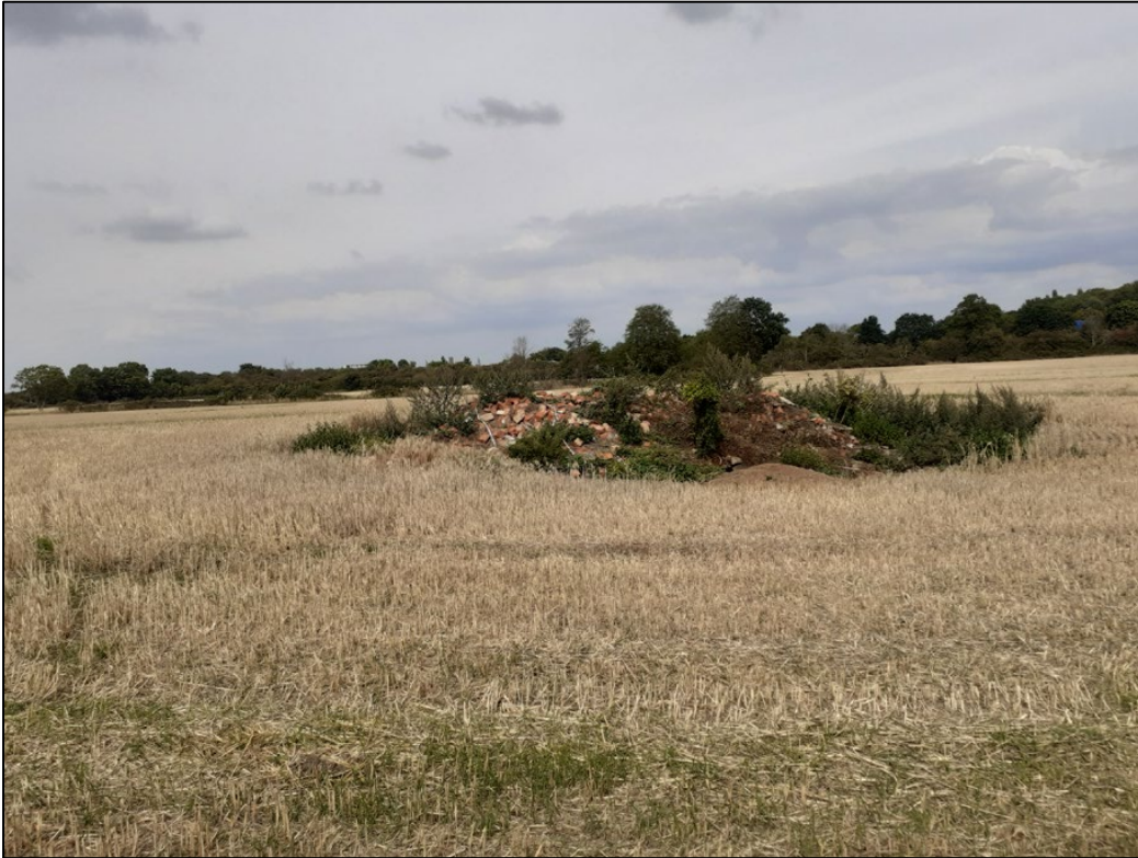
Plate 5: Collapsed structure in Area 21, looking north
